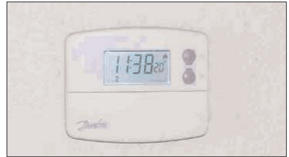
Danfoss 5000 TP programmable room thermostat
